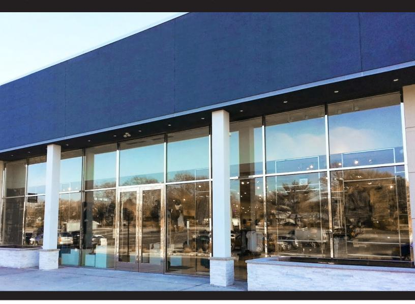
API's full range of Storefront Framing Systems includes systems such as the Industry Standard 2" x 4-1/2" Front/ Center-Set system for 1" glass (which is also available as a Thermally-Broken system), our exclusive 2" x 4-1/2" Center-Set system for 1/2" glass, and our 2-1/2" x 5" HVHZ Impact System. We can also clad our storefront systems in a variety of metals and finishes, such as polished stainless steel, oil rubbed bronze, brass, hot rolled steel, colored stainless steel and more.
